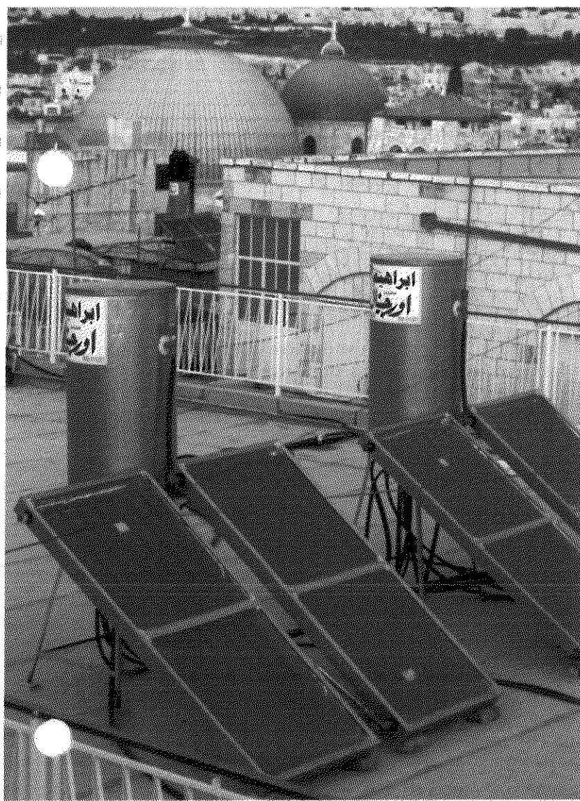
▲ FIGURE 9-48 SOLAR PANELS Solar panels installed on apartment rooftops in the Old City of Jerusalem are used to heat water, which is stored in the adjacent tanks. The domes are the Church of the Holy Sepulchre, built at the site where Jesus is thought to have been crucified, buried, and resurrected (see Chapter 6).
