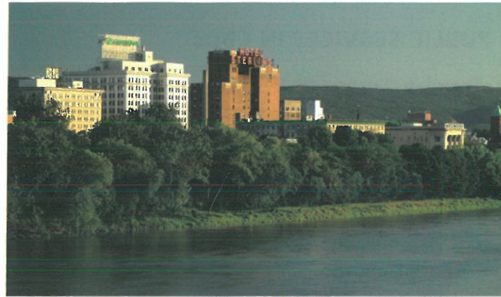
▲ FIGURE 13-3 SITE OF WILKES-BARRE'S CBD Wilkes-Barre was built along the south bank of the Susquehanna River.
